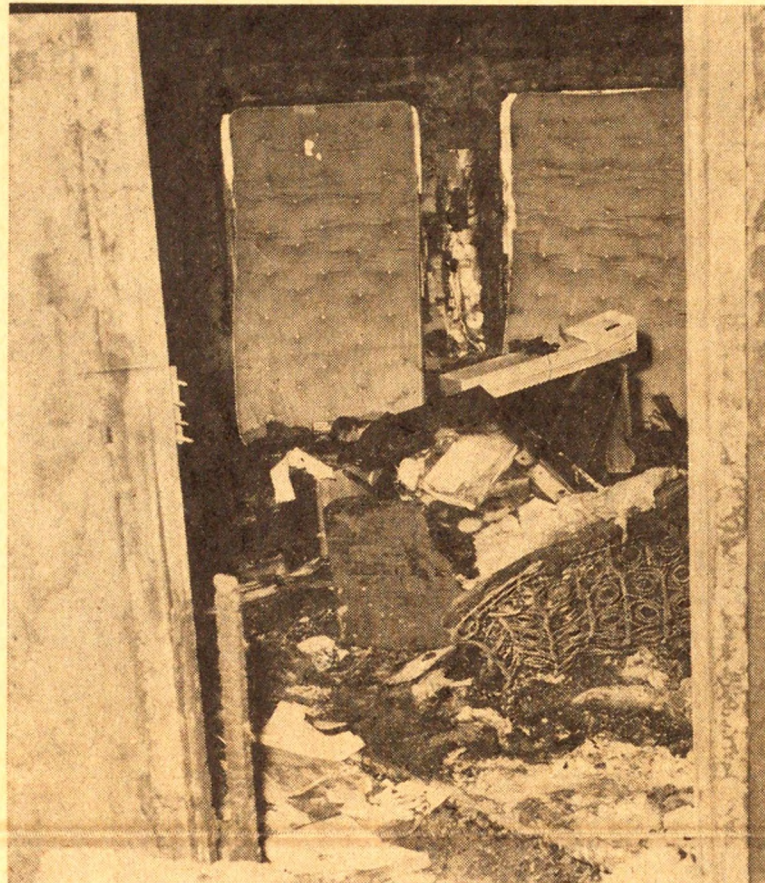
Above, is the debris that remains of a room at Siena Heights College, Adrian, Michigan. The mid-March fire, swept through the fourth floor of Ledwidge Hall.
