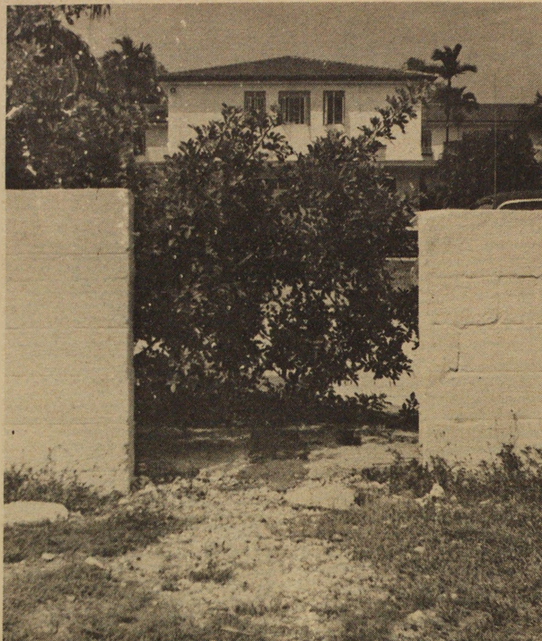
The above photograph was taken along the wall in front of Dalton-Dunspaugh. Previously, this opening was a throughway for pedestrians and cyclists, but shubbery has now blocked the passage way. Hopefully, in the near future, this problem will be corrected and no parking signs erected so that the passage will again be useful.
