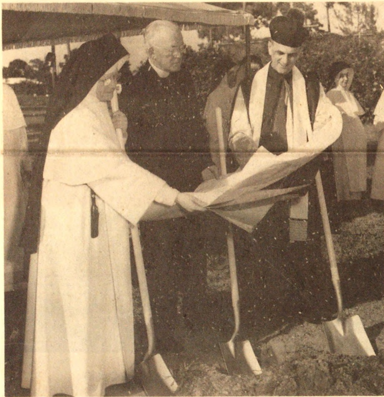
Ground-breaking for Fine Arts Building and Auditorium, 1954. From left to right: Sister Mary Edmond, Monsignor William Barry, Monsignor George Rockett.
