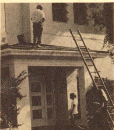
$85,000 spent renovating roof. Photo Randy Sidlosca
