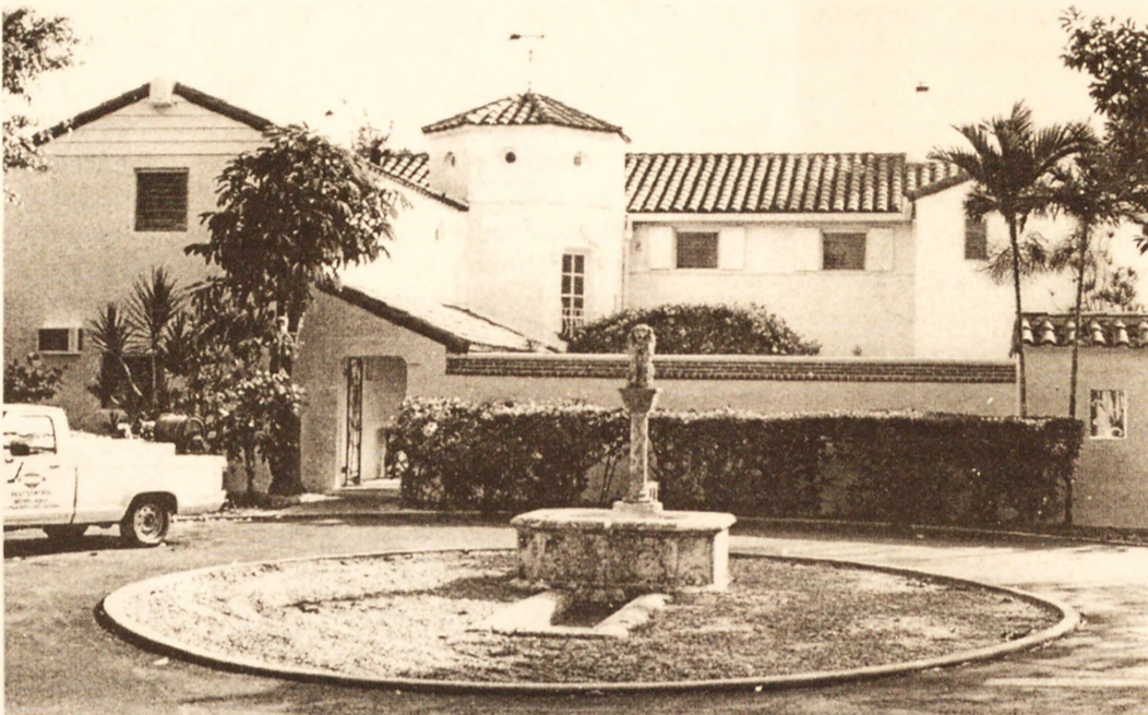
The Miami Beach house needed plumbing and wiring when Sr. Jeanne moved there in 1987
