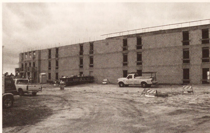
New residence halls currently under construction at Barry University.
