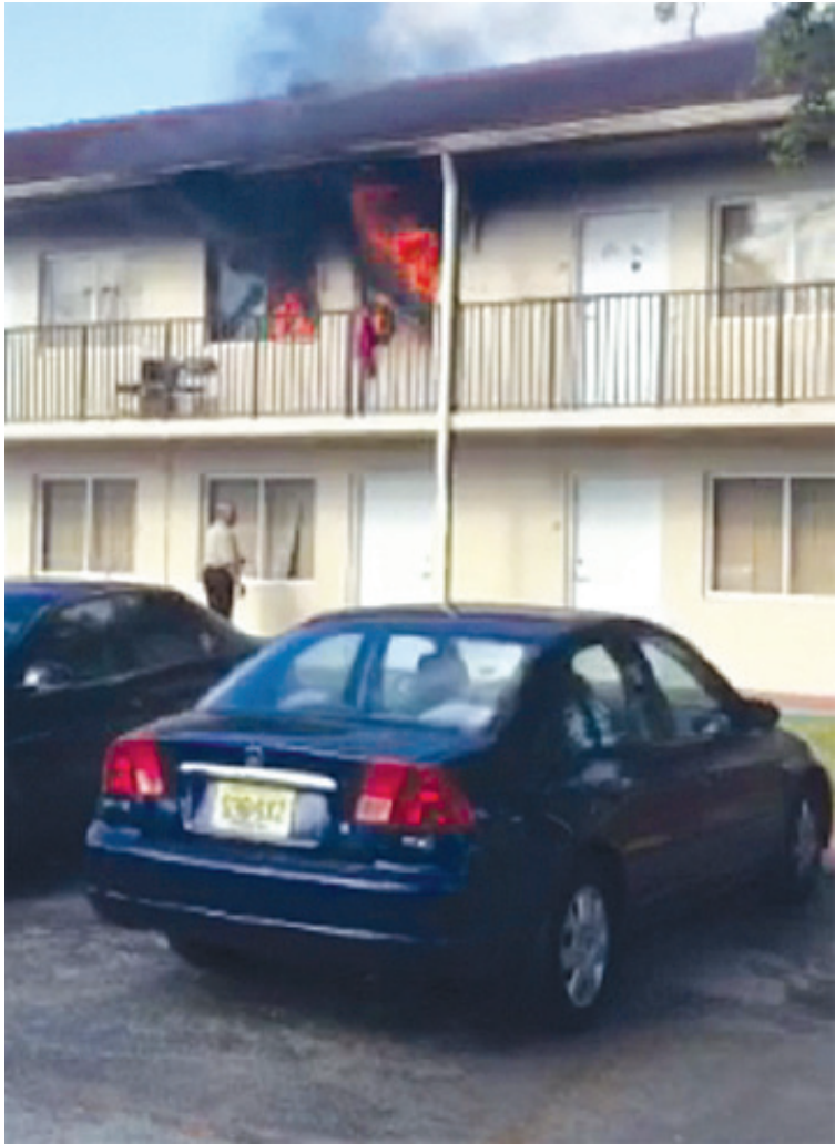
A fire in Browne Hall on April 7, damaged six rooms. For more about the story, turn to Fire in the Hole on page 2.
